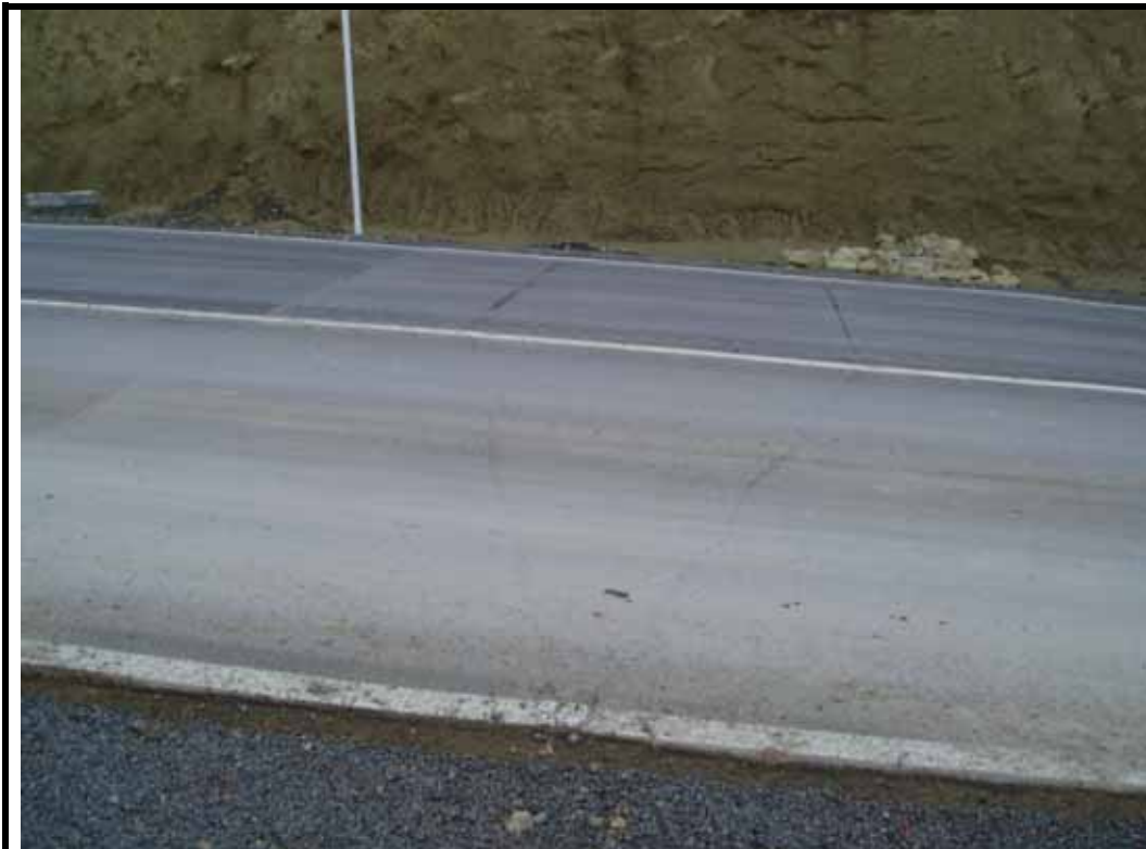
Description: Peek counter / classifier on LAR. The piezometer tubes are in the downhill(outward) lane.
