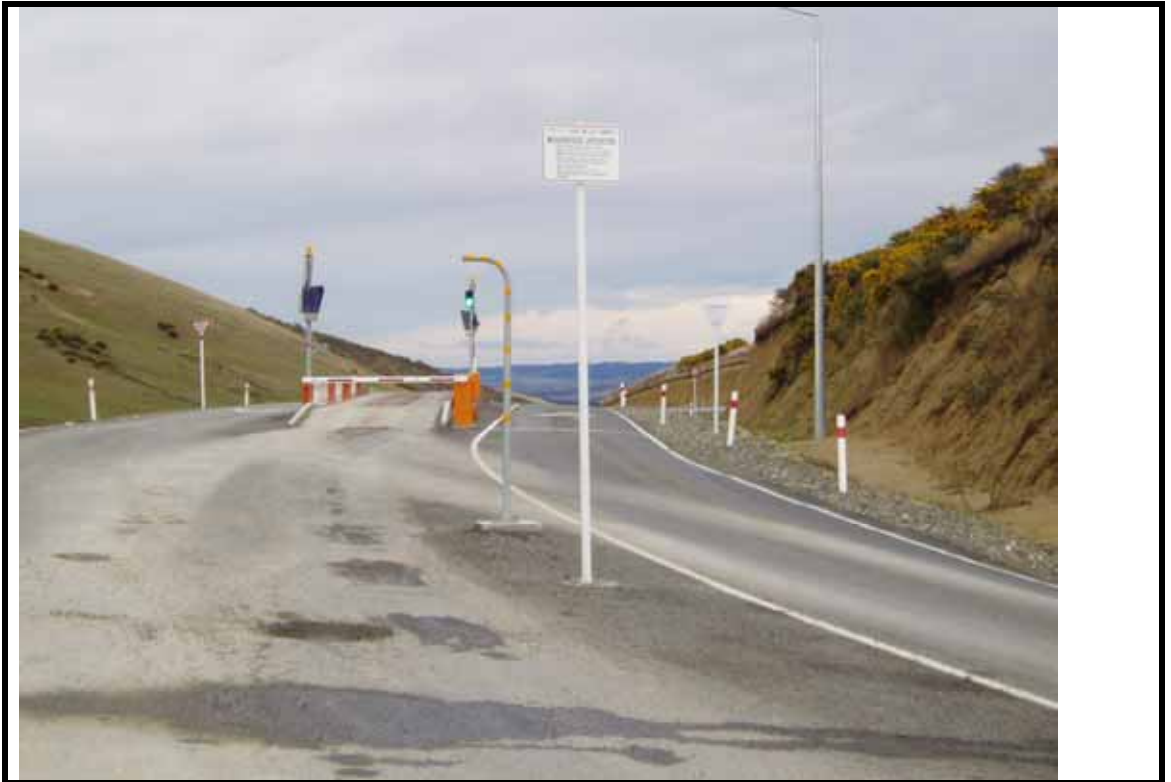
Description: Automated weighbridge on LAR. The weighbridge can only be accessed by vehicles that are issued with a Dallas tag. The tag reader is mounted on the pole in the foreground.
