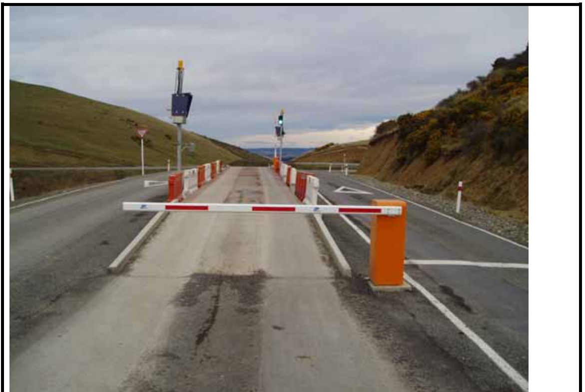
Description: Automated weighbridge on LAR. The weighbridge can only be accessed by vehicles that are issued with a Dallas tag. The console on the LHS is used by vehicles when leaving the landfill.
