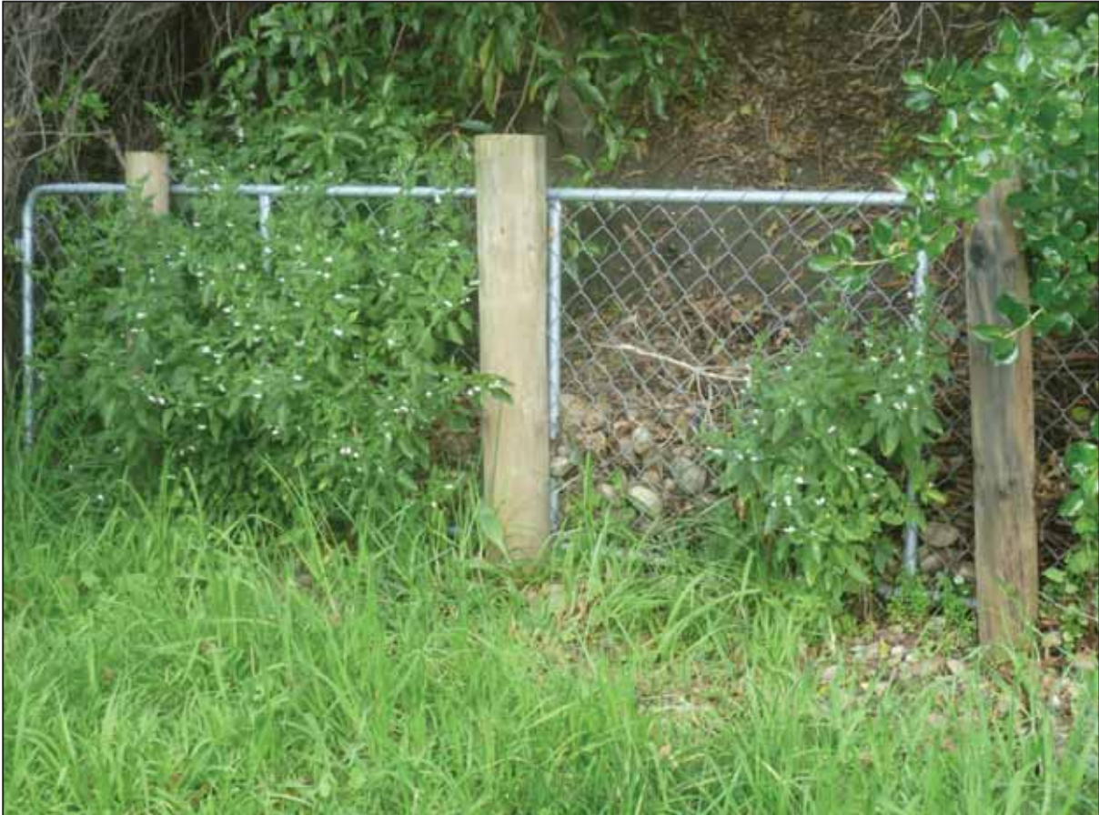
Photo 1: Rockfall protection barrier installed by campsite manager
