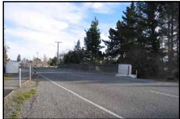
Bridge on northern side
