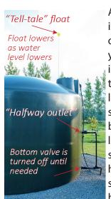
Another great idea is installing a halfway outlet. This enables you to use the water in the top half, and then if you accidentaly leave a hose on, or stock knock off a ballcock you will not lose your entire water storage. If this does happen you and switch to the bottom half
