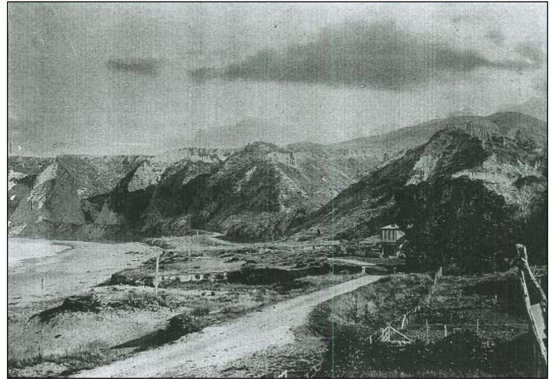
Looking south before the school was built
