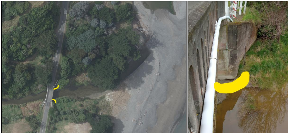
Figure 8: Protection of Buxton Creek Bridge abutments
