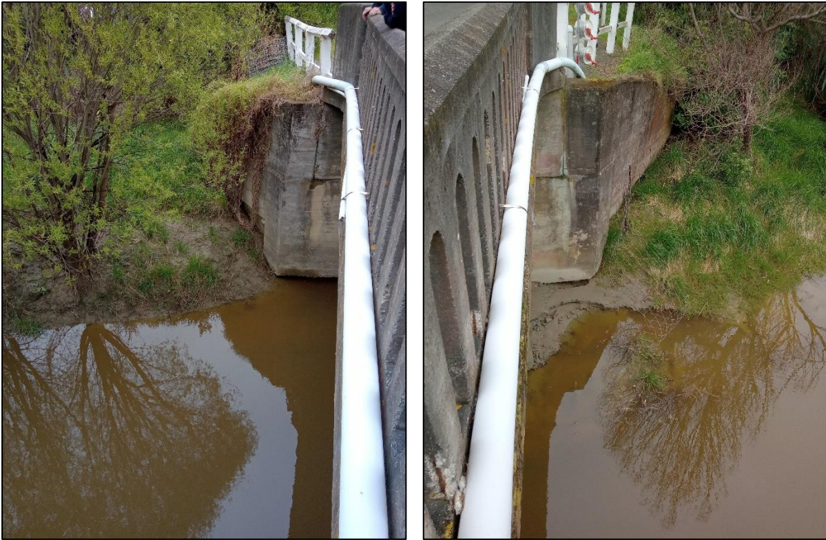
Figure 5a and b: Buxton Bridge downstream abutments
