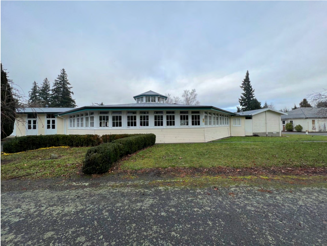
Figure 16 North west corner
