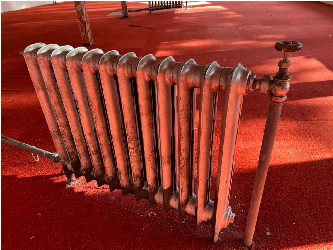
Figure 31 Original cast iron radiator
