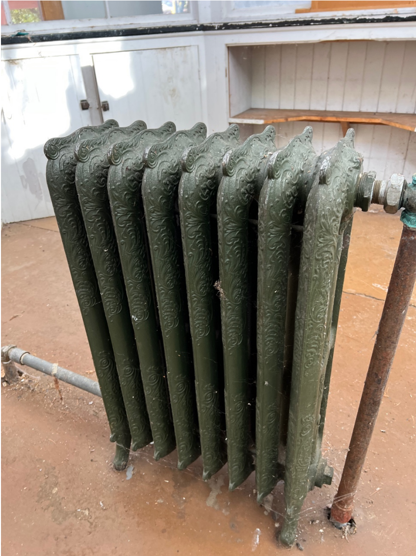
Figure 30 Original cast iron radiator
