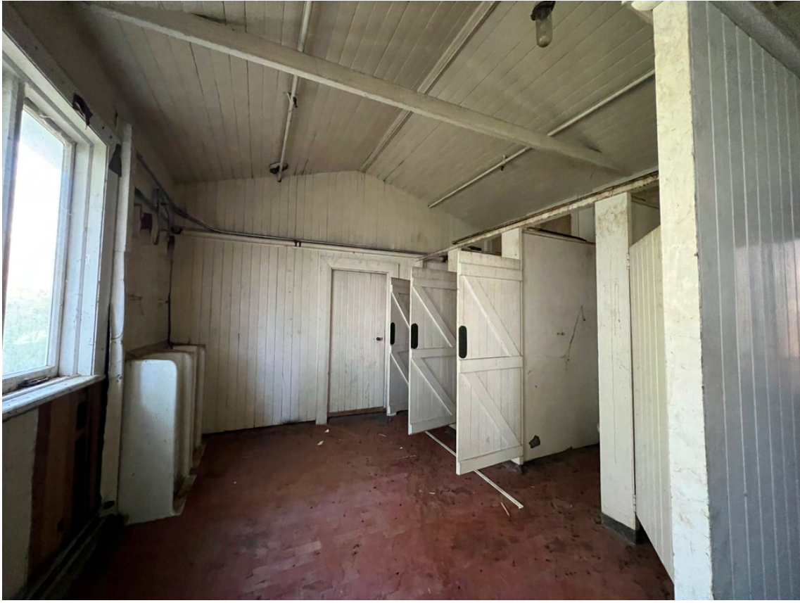
Figure 33 East wing toilets
