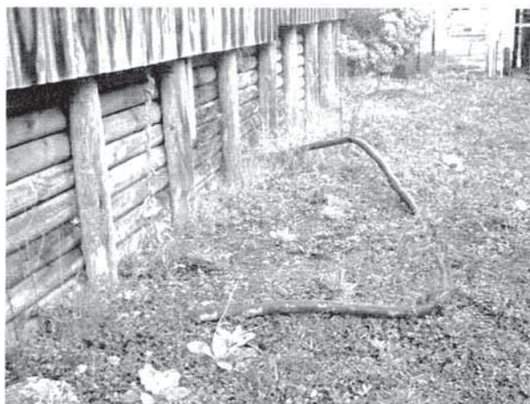
Figure 15: Gas pipe remains, possibly from main pool (© Author, 2004).
