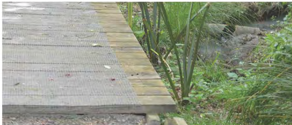
Small timber bridges, steps and compacted gritted paths across Hospital Stream
