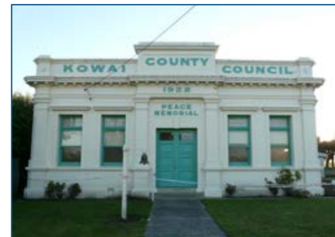
Kowai County Council Chambers
