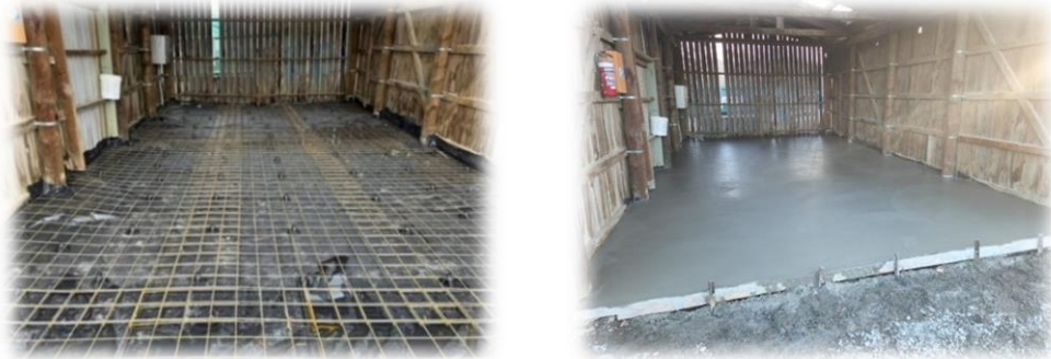
Hanmer Springs transfer station shed floor pre-pour and post-pour.
