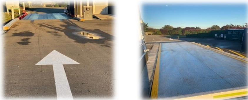
New weighbridge and site direction markings
