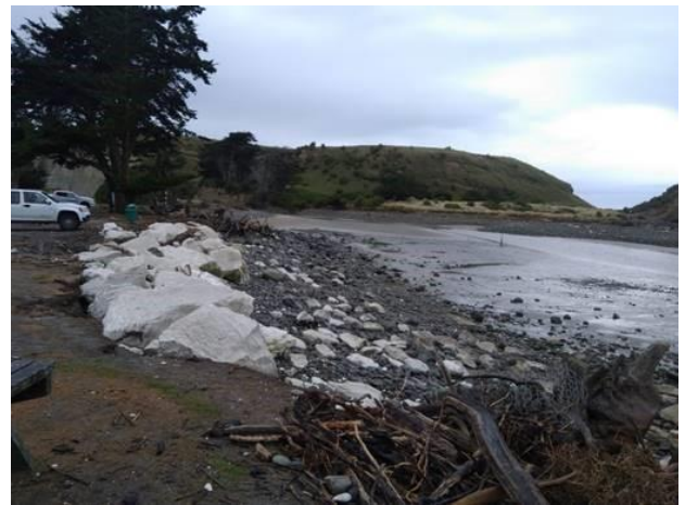
Figure 5.3: (a) Erosion of Motunau high coastal cliffs; (b) Motunau River lower terrace - bank armour rock protection immediately upstream of the river mouth.
