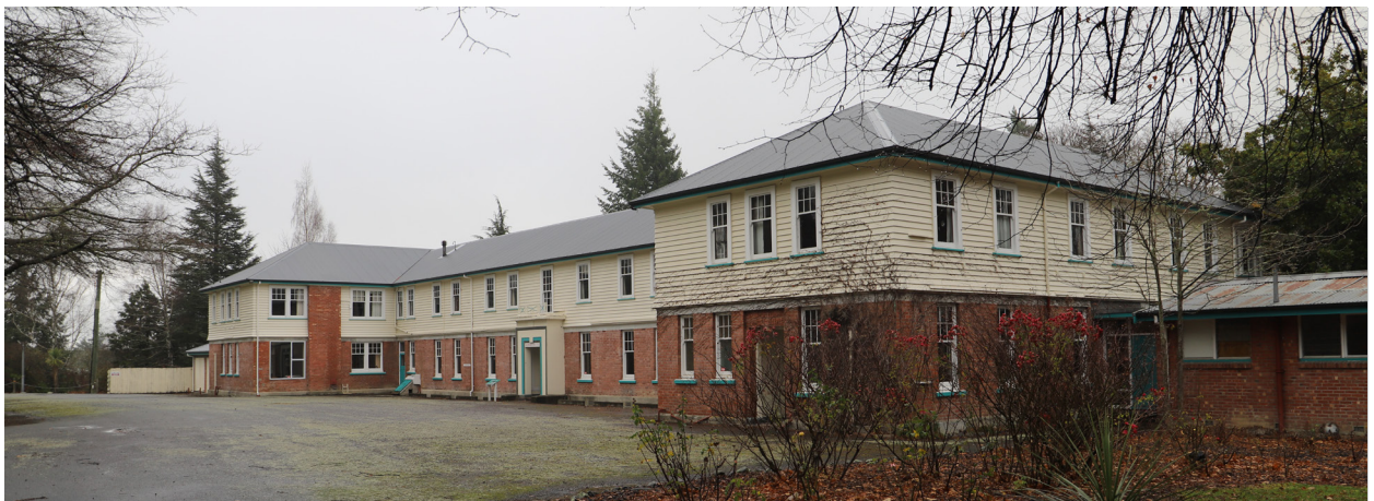
Photo 11: While the buildings within the Queen Mary Hospital site depict a number of different architectural periods, the colour of all the buildings is light yellow/ cream with white trims.
