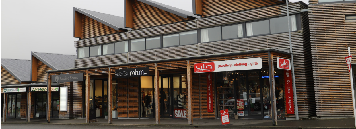
Photo 8: The sawtooth roof form is a contemporary response to the required roof angle that breaks up the built form.
