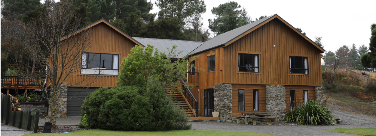
Photo 1: An example of a contemporary interpretation of the alpine character with board and batten cladding and use of riverstones. Recessive, natural colours blend the building into the landscape.
