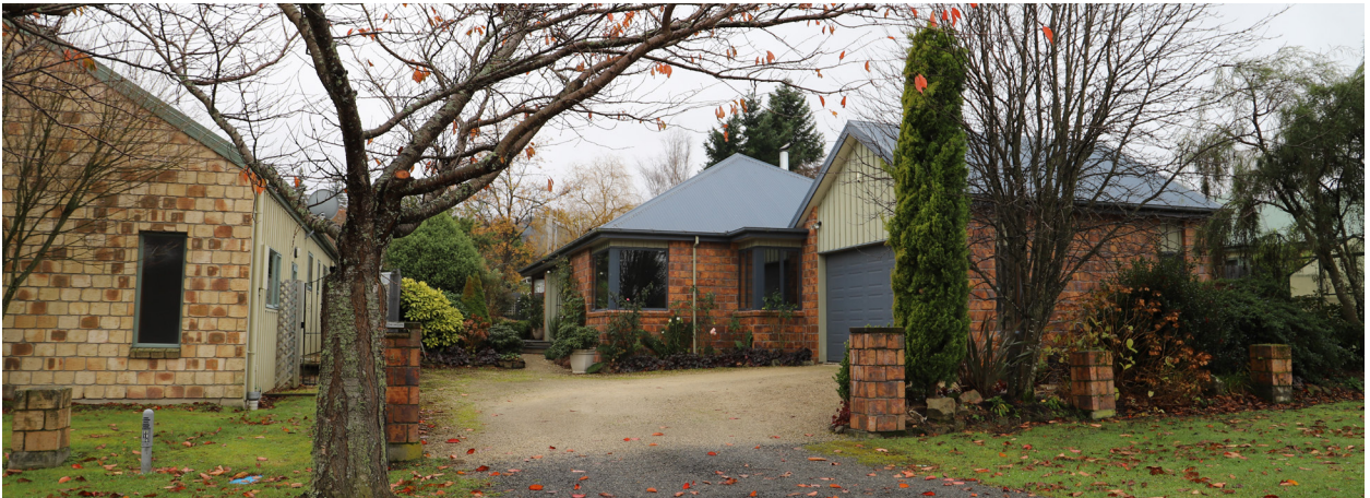
Photo 6: The buildings along the northern side of Bath Street do not support the heritage character of the Old Town area. It is recommended to reduce the Old Town Design Area and confine it to the terrace edge between Bath Street and Leamington Street.
