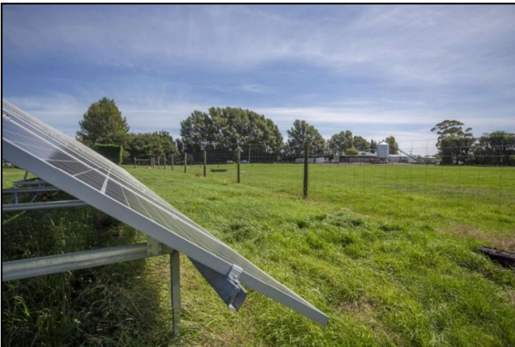
Figure 11: Another NZ Solar Farm - Keswick Farm Dairies Ltd, Rangiora. The photo shows grass coverage over the ground does not diminish because of the PV modules.
