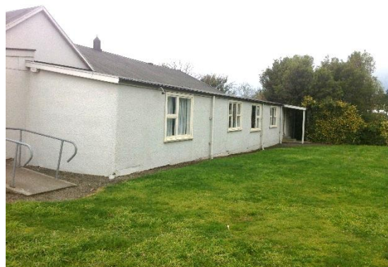
Photo 2 – View of rear elevation
