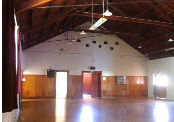
Photo 4 – View to inside of north elevation of main hall (timber internal wall).
