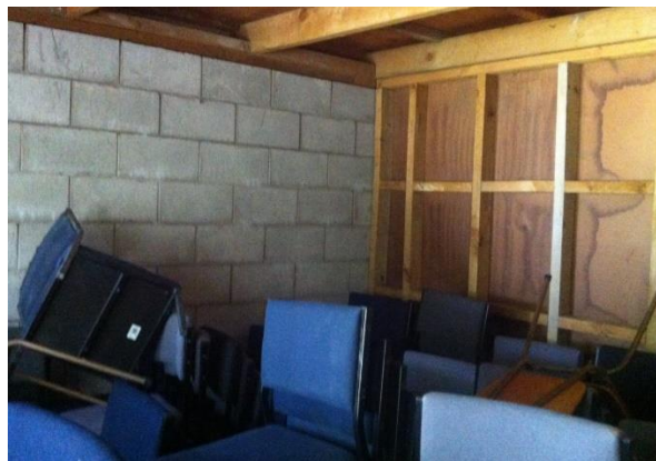
Photo 6 – Internal view of western blockwork extension.
