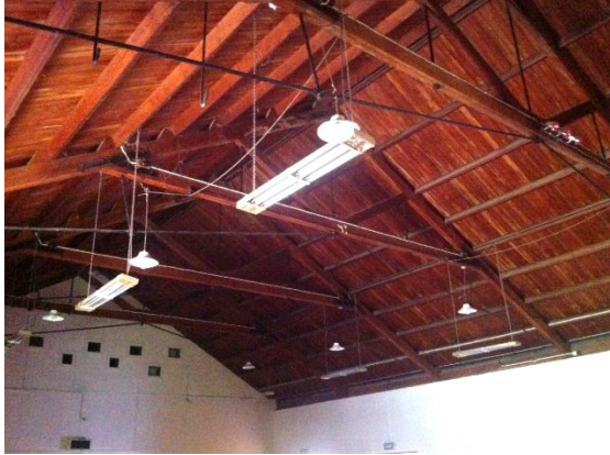
Photo 3 – View to underside of main hall roof.
