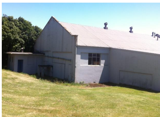
Photo 2 – View of rear elevation
