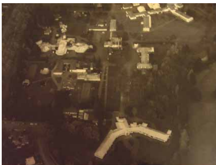
Digital photograph of an aerial photograph of Queen Mary Hospital Site displayed on the wall of the Maintenance Engineer's Office, dated 1966, RNZAF, from Opus Report
