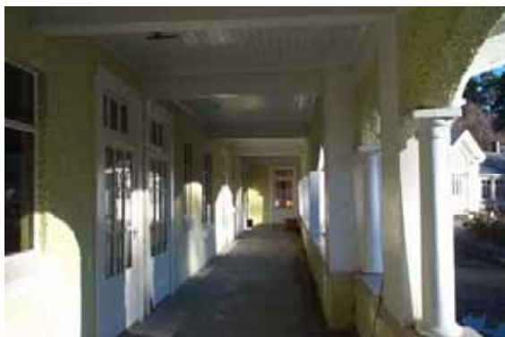
Open verandah on north elevation of east 'butterfly' wing, June 2004.
