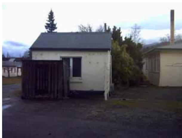
Detached brick building to the south of the Soldiers Block. Possibly the meat safe/dairy from the early 20 th century?
