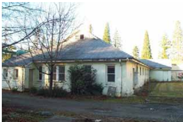
Gymnasium, west and south elevations. Photo June 2004.
