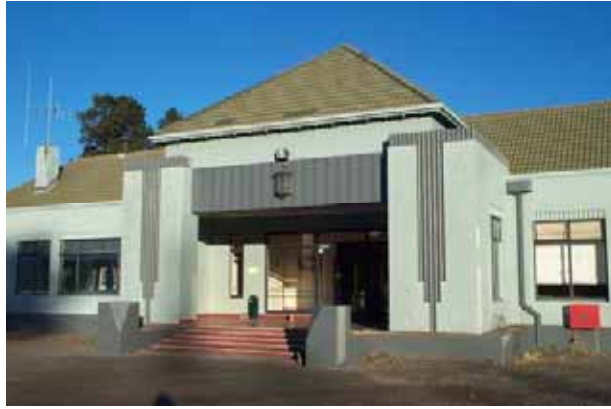
Main entrance Rutherford Block, on north side.
