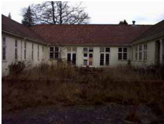
Fountain House (with fountain at centre of courtyard), photo taken from the north, June 2004
