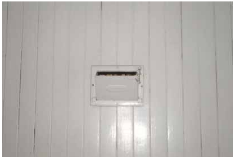
Ventilation opening on interior (tongue in groove) wall of Morgue
