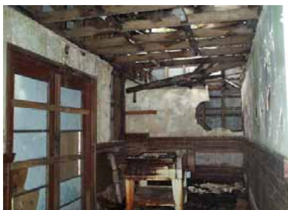
Dog-leg corridor from Gymnasium Building going through to Fountain House, June 2004.
