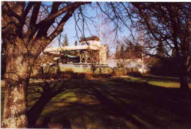
The industrial looking and 'wild' hydroslide aspect of the pools visible rising up some height above the top of the fence line. This has a negative effect on the character and ambience of the Queen Mary site. (Identity area 1)
