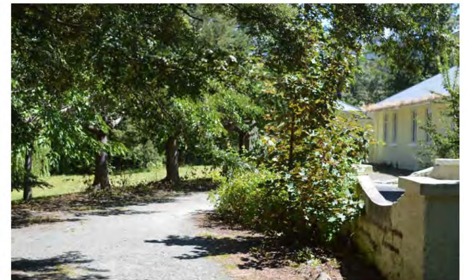
Photograph 18. South Chisholm Ward overgrown and neglected
