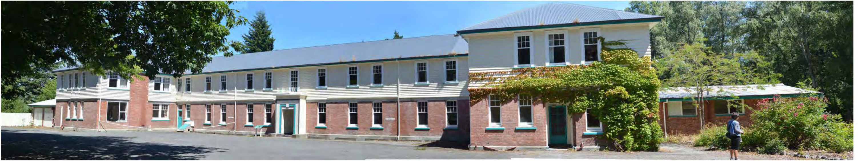
Photograph 26. Nurses Hostel frontage - looking west
