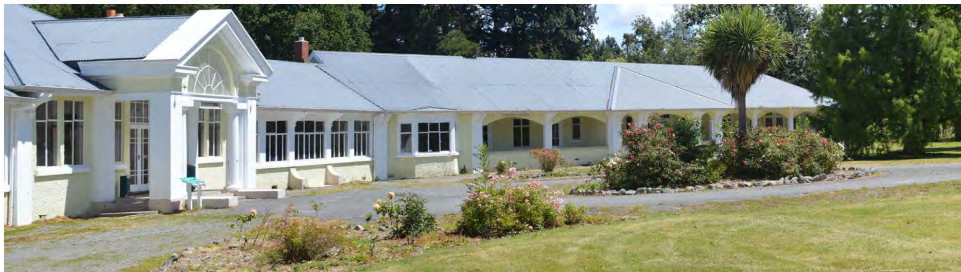
Photograph 12. Chisholm Ward frontage looking east
