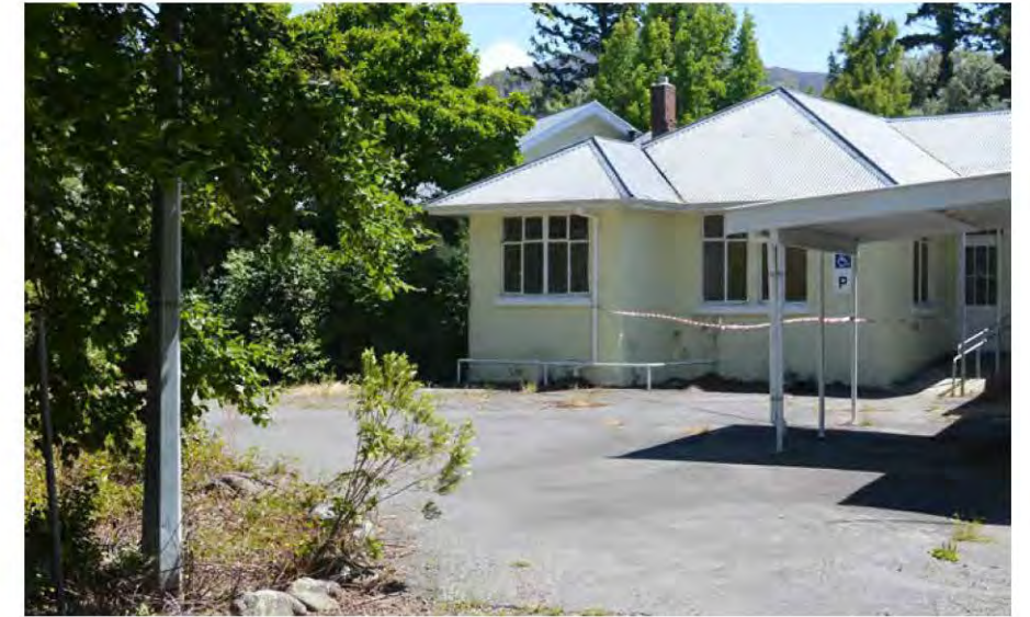
Photograph 15. South Chisholm Ward overgrown and neglected
