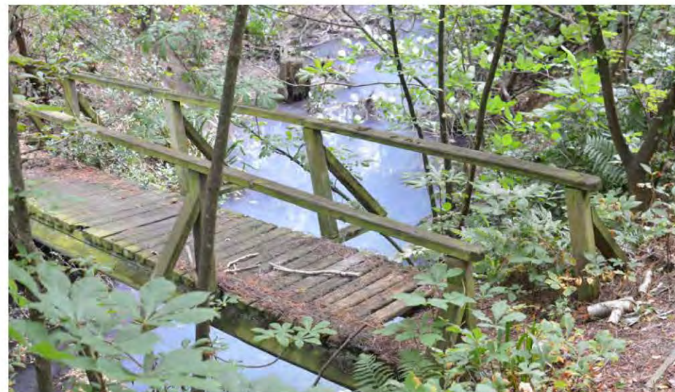
Photograph 40. Derelict footbridge to southwest of boundary
