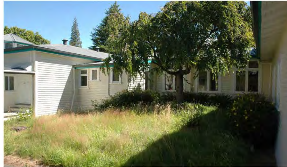
Photograph 38. Internal garden space at the back of the Soldiers Block
