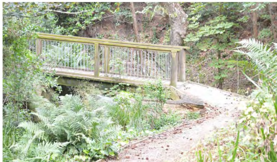
Photograph 6. Hospital Stream footbridge
