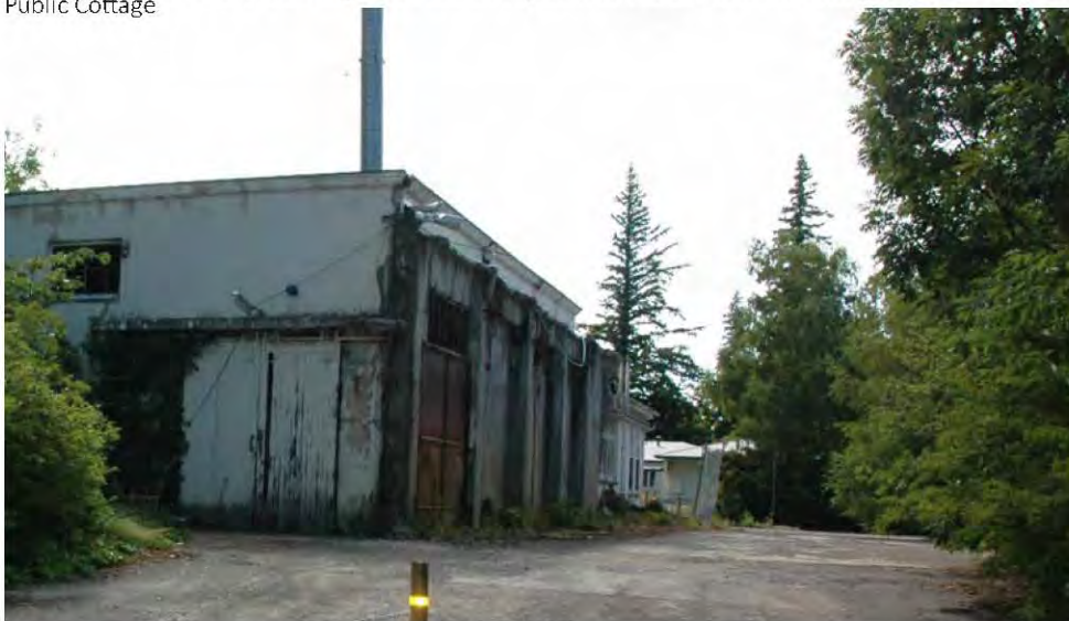
Photograph 42. Derelict buildings to come down just inside southern boundary of site
