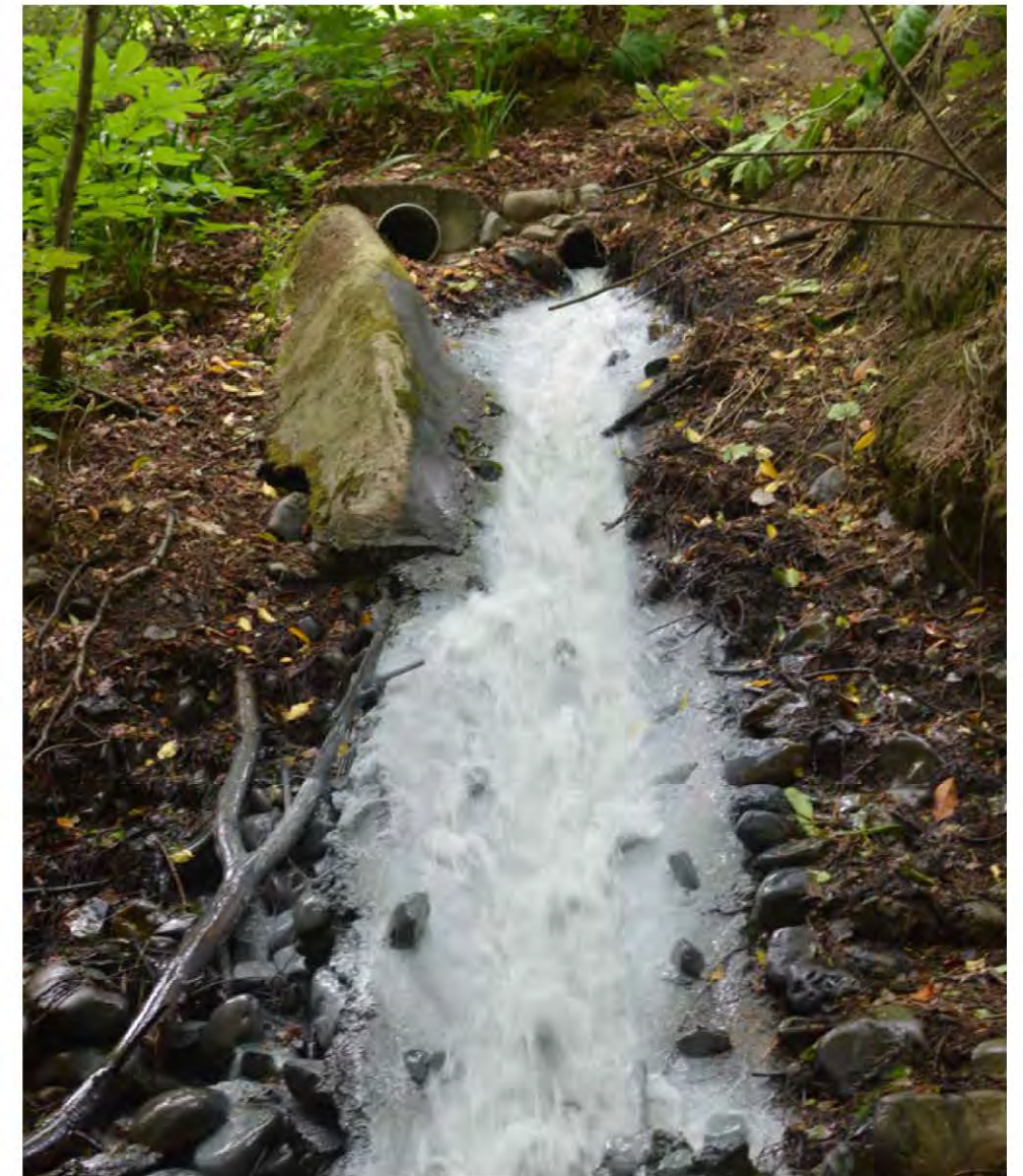
Photograph 7. Thermal discharge into Hospital Stream
