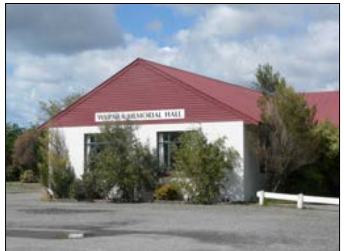
Waipara Memorial Hall
