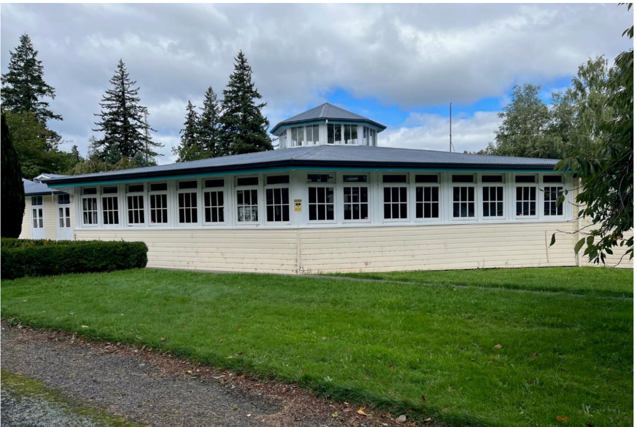
Northern elevation of western ward
