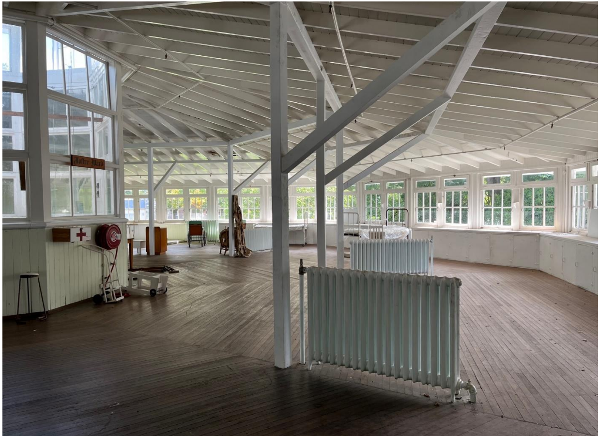
Figure 5: Western octagonal ward. March 2023
