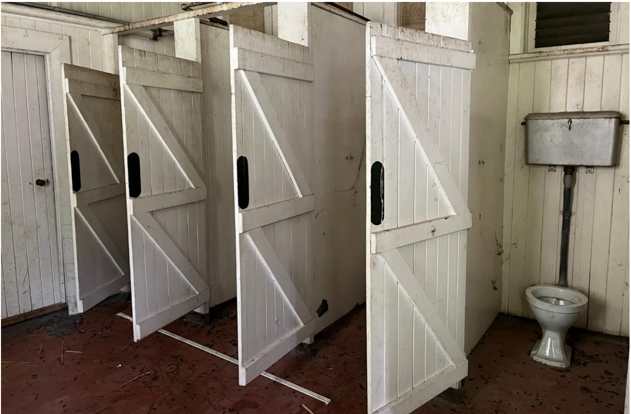
Original toilet block attached to eastern ward
