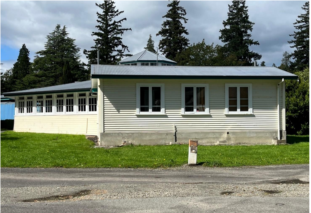
Toilet block to west of western ward
