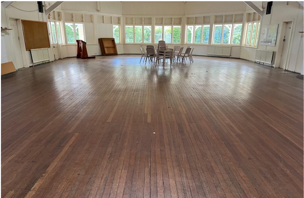
Floor of Dining Hall
