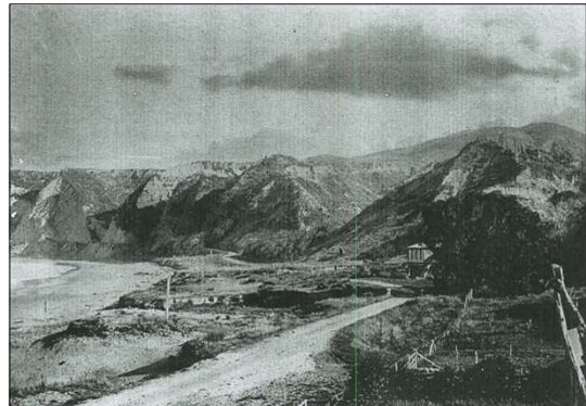
Looking south before the school was built
