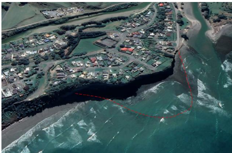
Figure 4.5: Approximate shore platform area where rocks would be sporadically placed at a spacing of 1 every 4 m 2 to break up wave energy approaching the cliff toe.
