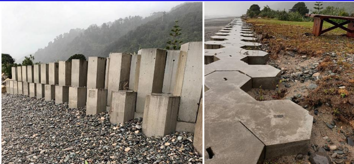
Figure 4.4: (Left) front view of Westlock interlocking concrete wall design; (right) top of interlocking concrete wall structure. Photos sourced from: Westlock Ltd.
