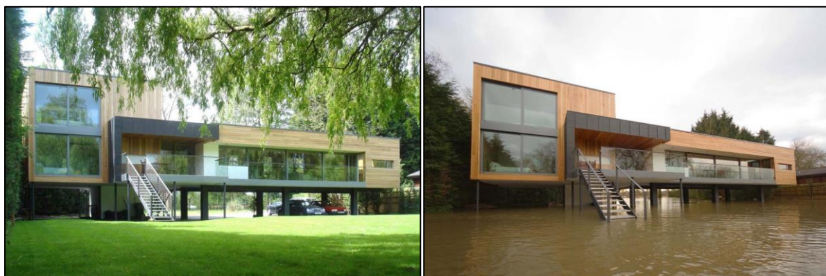
Figure 2a and b: Raised dwelling to cater for flood waters 8
