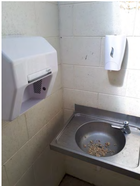
Figure 8.7b Wide-angle view of above. Water will not drain away when basin is used for its intended use. It is the only handbasin in the mens toilets. Toilet users have told us there have been Freedom Campers washing dishes in the handbasin, while they used the urinal immediately adjacent.
