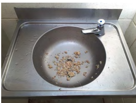
Figure 8.7a Porridge blocking hand-basin in mens public toilets adjacent to Freedom Camping area.
