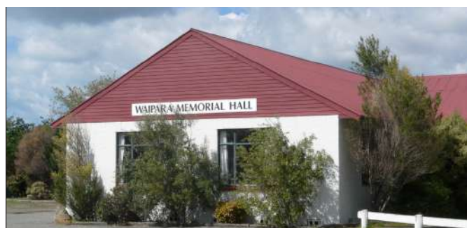
Waipara Memorial Hall
