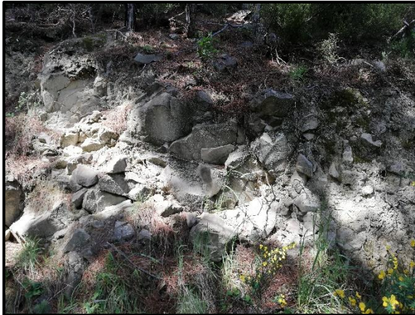
Photo 3: Example of highly fractured rock that is exposed near the surface
