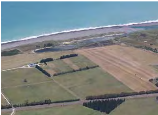
The river mouth is deflected to the north of the river channel by drifting beach sediments.
