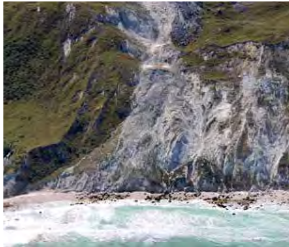
Southern base of Montserrat Earth Flow.
