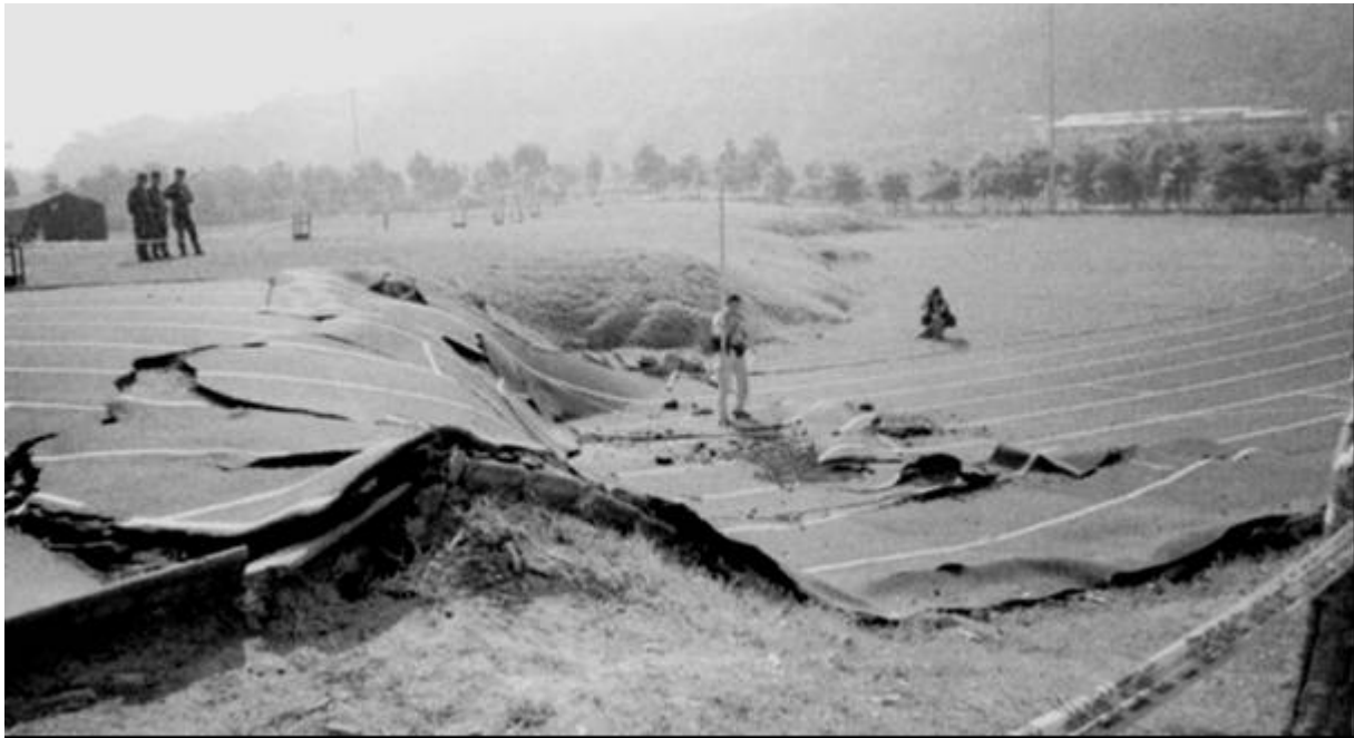
Figure 10 Fault scarp formed on the Chelungpu Fault during the magnitude 7.6 Chi-Chi Earthquake, Taiwan, 1999. The disrupted running track shows damage typical of a reverse fault ground-surface rupture, which is well expressed on the brittle surface (note the smoother rupture across grass behind). This location lies on a stream terrace that is younger than the previous rupture event on the fault, so that there was no scarp here before the earthquake. This example illustrates the sorts of effects that can be expected on active reverse faults of the Hurunui District the next time any particular fault experiences a surface rupture earthquake. Photo and information from Kelson et al. (2001).
