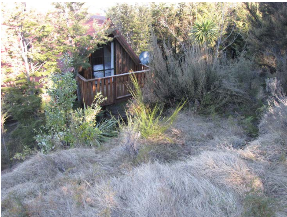
Figure A1.10 Arcuate slope cracking (facing away from view angle) and ground failure (in foreground) above a cut slope at a property on Charwell Terrace.
