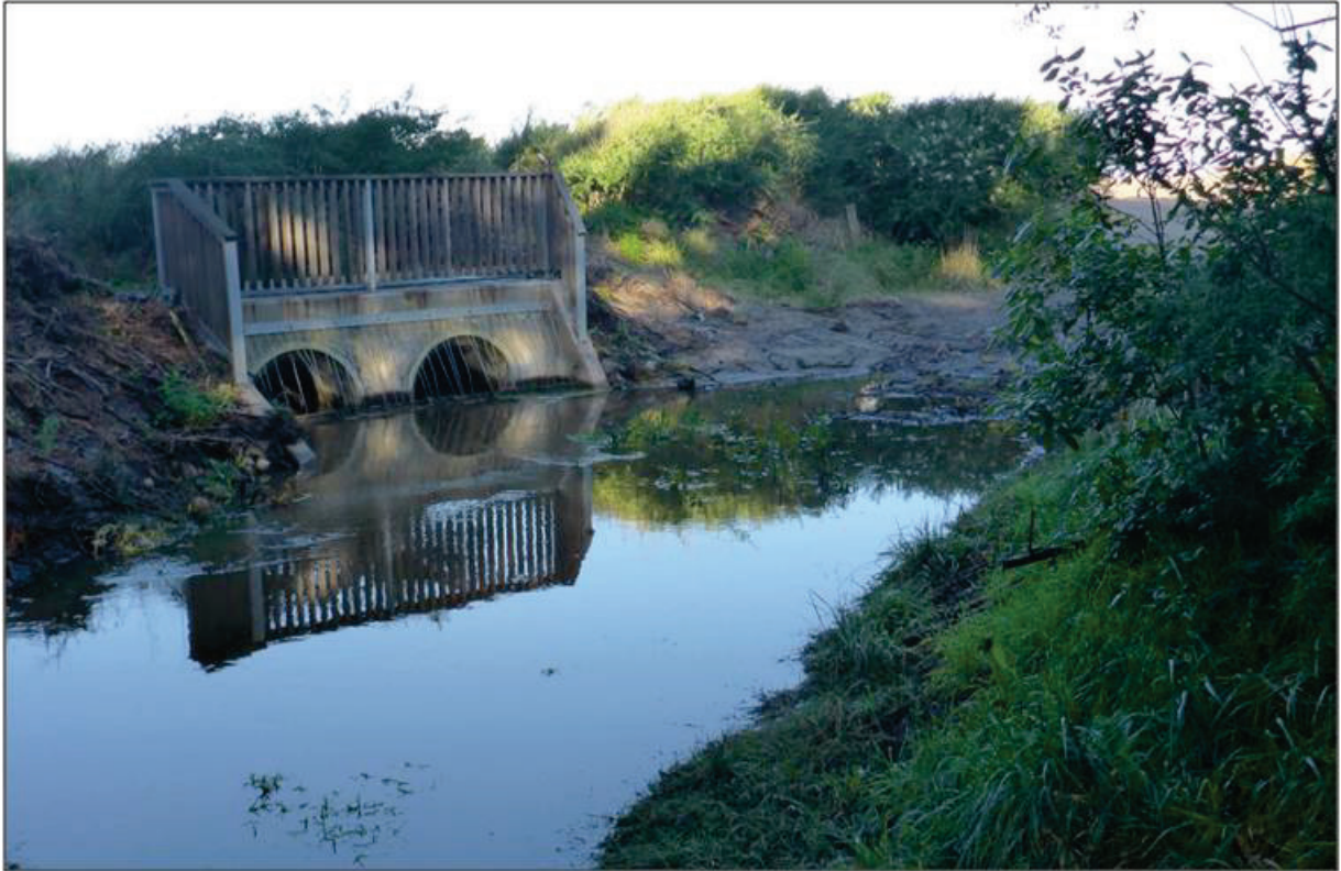
Figure 2-13: Leithfield Outfall Drain piped outlet to the sea - Inlet
