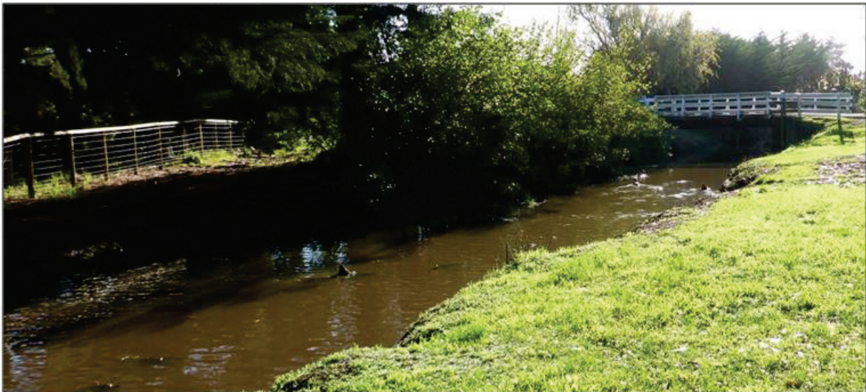
Figure 2-12: Leithfield Outfall Drain passing through Leithfield Beach settlement
