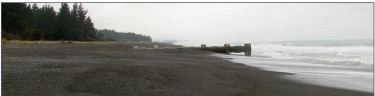
Figure 2-14: Leithfield Outfall Drain piped outlet to the sea - Outlet
