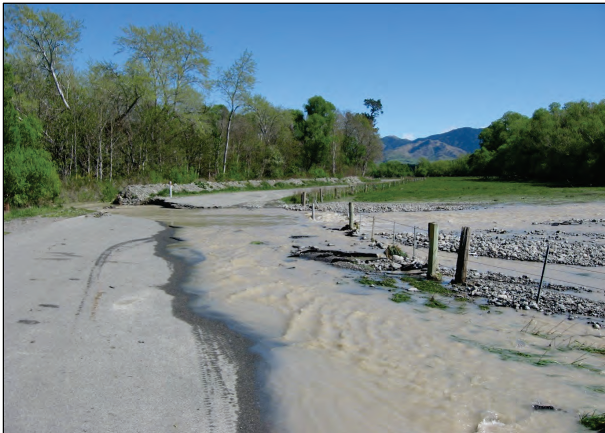
Figure 2-6: Looking west along River Road to the breakout from the Waiau River. Photo was taken on 9 October 2007 at ~10:30 am (Waiau River is estimated to have peaked at this location on 8 October 2007 at ~8 pm)
