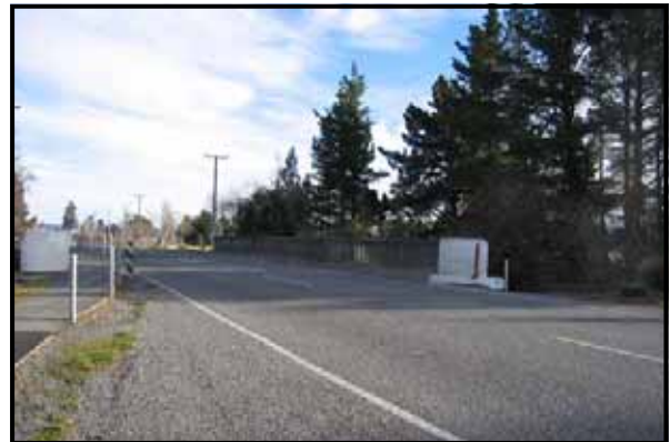
Bridge on northern side
