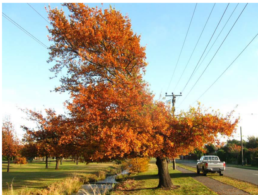
Large trees planted too close to high voltage power lines
