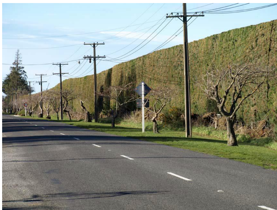
Small trees planted under low and high voltage power lines
